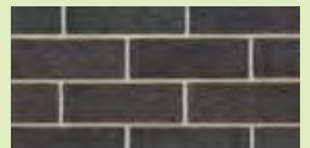
Natural colour mortar with rolled joints
