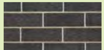
Natural colour mortar with rolled joints
