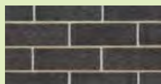
Natural colour mortar with rolled joints
