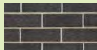
Natural colour mortar with rolled joints
