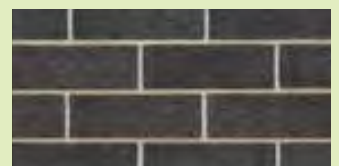
Natural colour mortar with rolled joints
