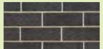
Natural colour mortar with rolled joints
